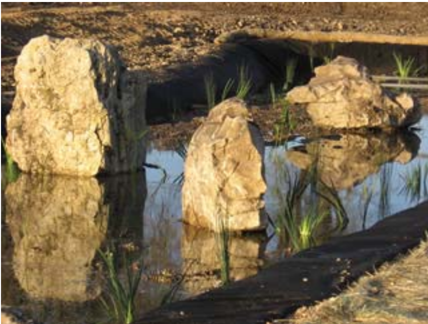
The completed upper pond.
