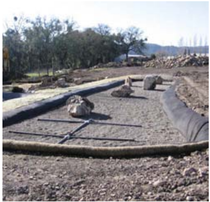
The upper reed pond, under construction
